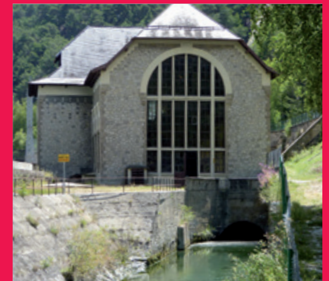
EDF's Combe d'Avrieux hydropower plant in the Alps, France
