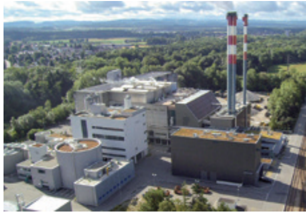
KEBAG waste-to-energy plant, Switzerland
