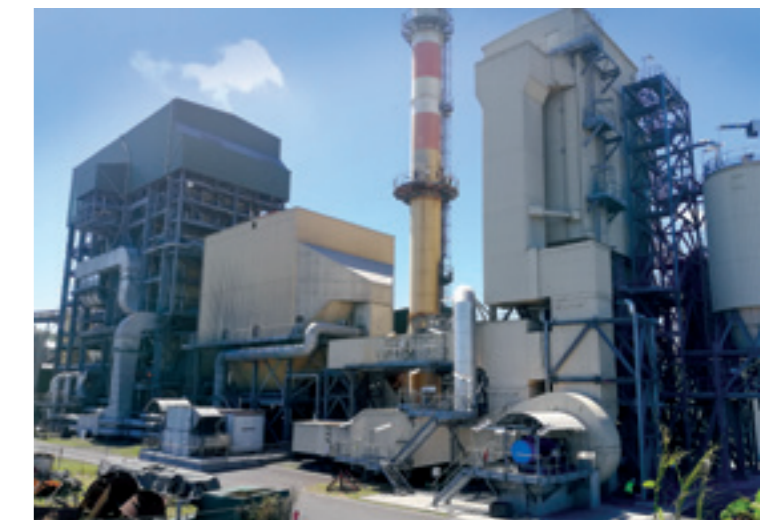
Bois-Rouge waste-to-energy plant on Reunion Island
